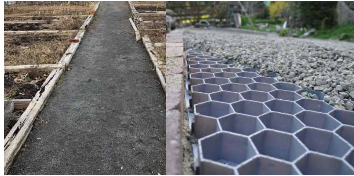
STONEDUST PATHWAYS, REINFORCED WITH GEOGRID
